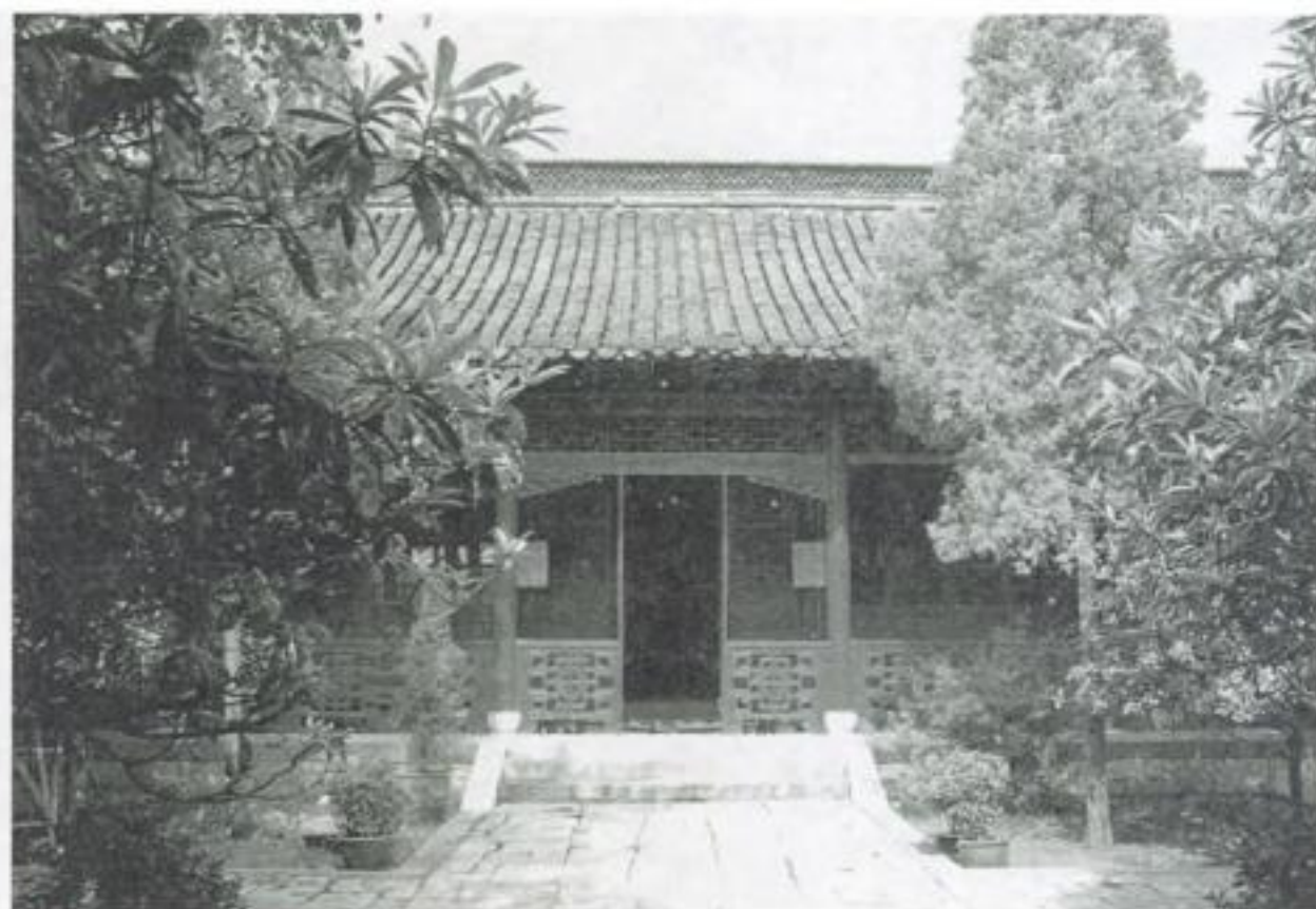
© Exterior of Zhenjiang Mosque.
